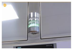
A beacon light and an acoustic alarm providing a quick audible and visual assessment of operation and failure states for the user.
