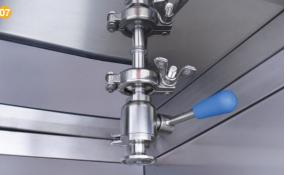
For outlet of liquid waste originating from sterility testing. Connection to a collecting tank or central waste.
